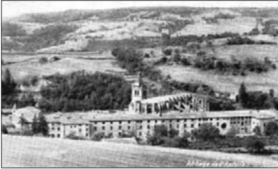
Abbey of Saint-Antoine. The Sisters’ part is to the right of the wheel-window.
