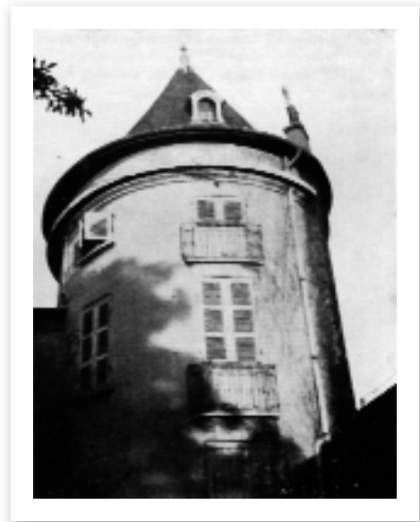
La Tour de Fourvière, Pompallier's residence
