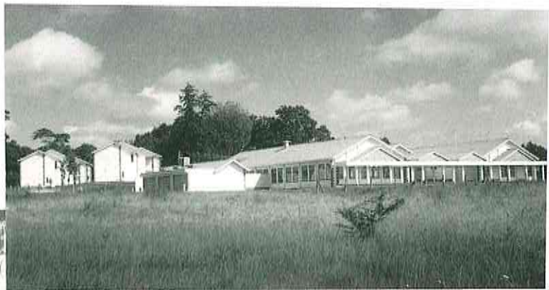
Partial view of the new buildings.
