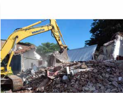
Mexico: Demolition of the Marist house of Asunción Ixtaltepec, Oaxaca
