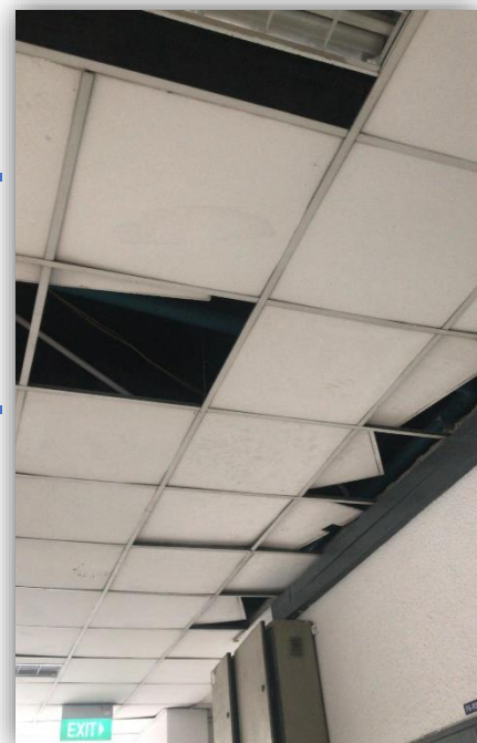
Block F level 5 and 6 ceiling boards were blown away.
