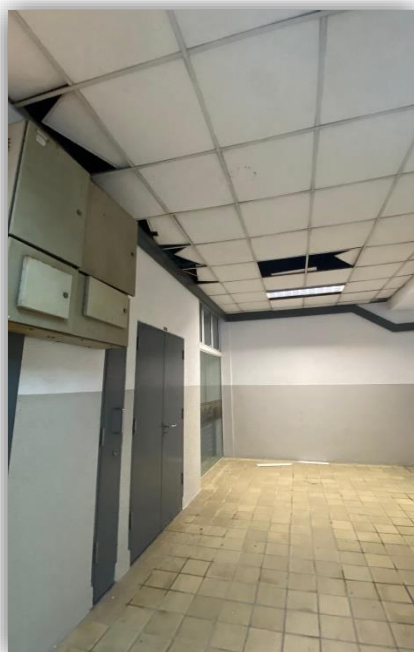
Block F level 5 and 6 ceiling boards were blown away.
