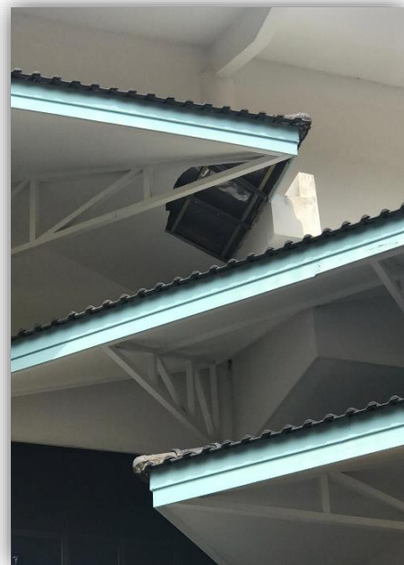
Ceiling of the chapel block collapsed
