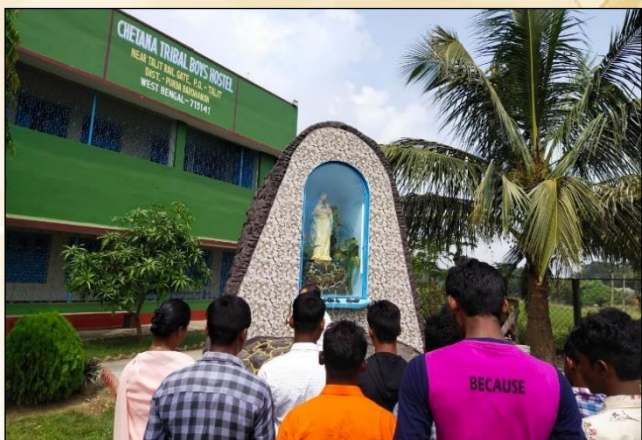
The Diocese of Asansol completed the renovation work of the hostel. Our hostel looks very new.
