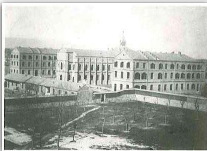
The Provincial House and House of Formation in Chala-Eul
